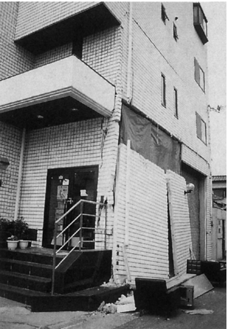
Figure 3. Ribbed ALC panels that fell during the Great Hanshin-Awaji Earthquake. The panels were of rebar-inserted longitudinal wall construction.
