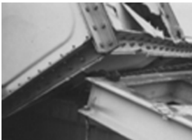
Figure 1. Anchor bolts came off
