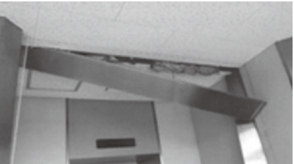
a) The ceiling finishing panel of an EXP. J has peeled off (photo: Satoru Ishiyama, Akita Prefectural University) 1)
