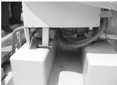
Figure 3. Deformation of the equipment's leg section
