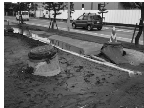
Figure 2. Raised manhole and cover (Urayasu City, Chiba prefecture)
