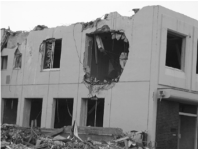
Figure 6. Exterior wall of relatively new reinforced concrete building which was destroyed by floating wreckage
