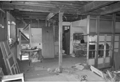
Figure 1. The state immediately after construction commenced. Construction started from the interior work leaving exterior walls as they were.
