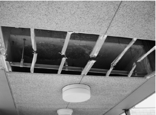
Figure 2. Ceiling materials at an expansion joint were broken and dropped off.
