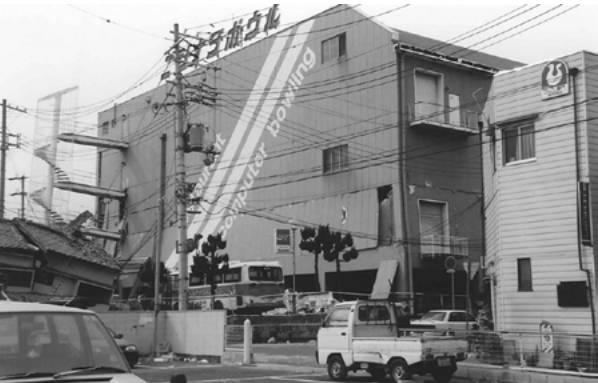
Figure 2. Collapse of an ALC panel (the Great Hanshin-Awaji Earthquake)
