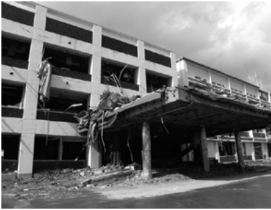
Figure 2. The City Hall of Rikuzentakata in Iwate prefecture suffered from flooding higher than the roof and was unable to function.
