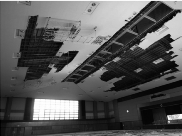
Figure 2. Ceiling collapse and damage at a gymnasium (the Great East Japan Earthquake, 2011) 1)
