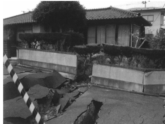
Figure 1. Damage to a valley filled building lot (Yamamoto-cho, Watari-gun, Miyagi prefecture, photo by Kazuya Mitsuji) 1)
