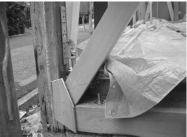
Figure 5. There are still many sub-standard seismic retrofit works.
