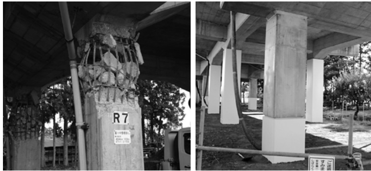
Figure 3. Damaged pier (left)2) and restored pier (right) (photo: both by Yoshikazu Takahashi, Disaster Prevention Research Institute, Kyoto University)
