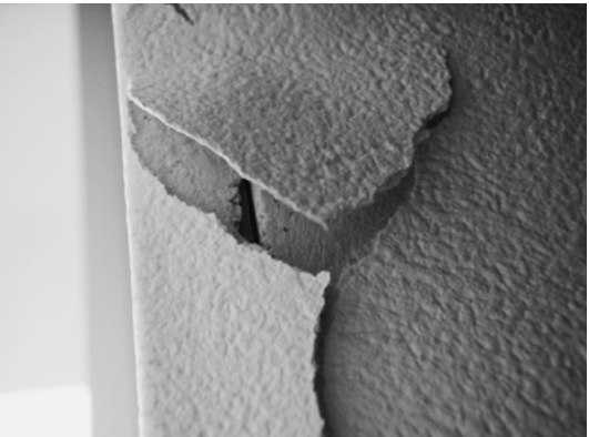
Figure 4. Partition walls with backings of light gauge steel in the hallway of super high-rise condominiums were broken.
