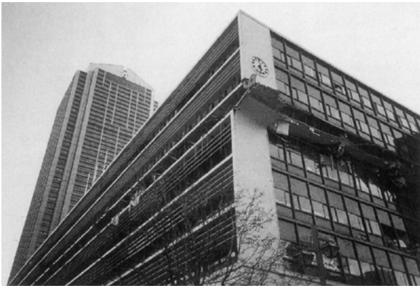
Figure 2. An example of the story collapse of an intermediate story 1)
