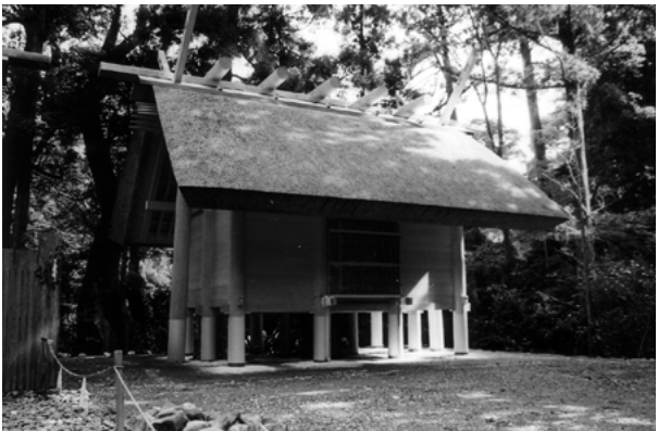
Figure 1. Shinmei-zukuri of Ise Shrine An architectural style with a raised floor and munamochi-bashira (ridge-supporting pillars) originated from a storehouse. Hafu (gables) supporting the roof penetrate and become chigi (forked roof finials).
