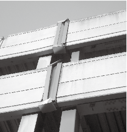
b) Deformation of a wall finishing panel of an EXP. J (photo: Tsuyoshi Seike)
