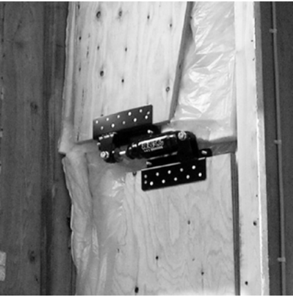
Figure 2. Seismic-response controlled structure using oil dampers
