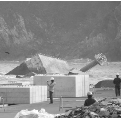
Figure 2. Broken seawall at Taro-cho The wall was overturned due to scouring at the base. In contrast, some seawalls and floodgates such as those at Fudai-mura, Iwate prefecture functioned with no damage.
