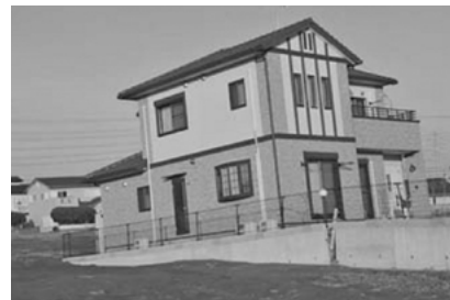
Figure 4. Inclination of a house caused by subsidence of land reclaimed from the sea (Fukushima district of Kamisu City, Ibaraki prefecture, photo by Koji Tokimatsu) 1)
