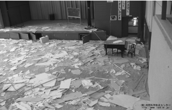
Figure 1. In this school gymnasium large amounts of ceiling materials fell off (the Great East Japan Earthquake, Sakae-mura, Nagano prefecture) 1)
