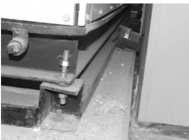
Figure 10. Deformation of the stopper due to misalignment of the vibration isolator
