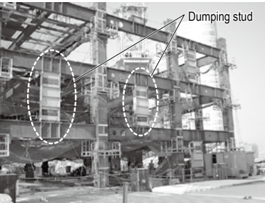
Figure 3. Vibration control stud
