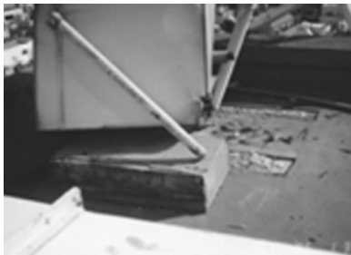
Figure 6. Overturning of beam-shape concrete foundation
