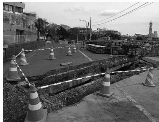
Figure 2. Difference of level caused by settlement of back filling under a bridge
