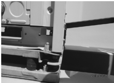
Figure 5. Deformation of vibration isolation base due to deformation of the equipment base member
