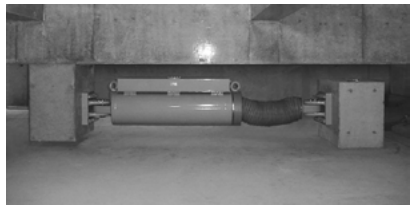
Figure 4. Hydraulic damper for base isolation
