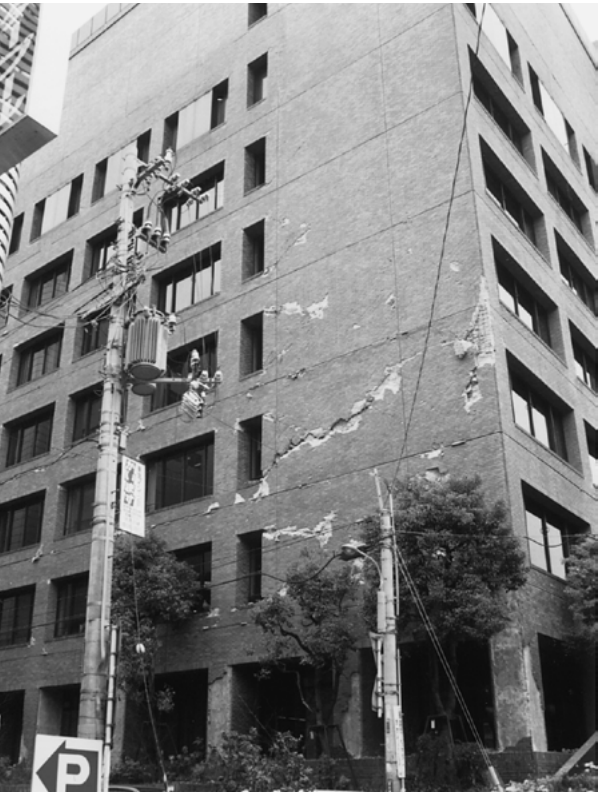
Figure 3. Damage to tile finishing which had been directly attached to the building frame
