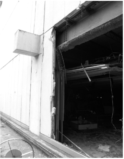
Figure 4. Damaged car park building for a commercial facility in Ofunato City, Iwate prefecture, caused by the Great East Japan Earthquake. Although the ALC panels suffered no damage from the earthquake, the tsunami broke through the wall and washed away the cars parked inside. This building was also of rebar-inserted longitudinal wall construction.
