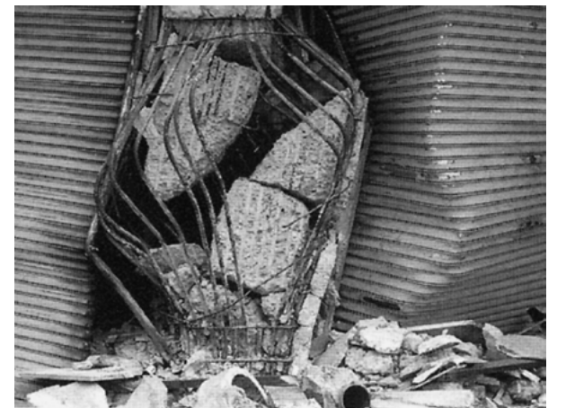
Figure 2. Hoops with spacing of 30 cm before 1970 (photo by: Faculty of Engineering, Tokyo Denki University) 1)
