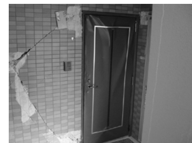
Figure 4. The entrance door has out-of-plane deformation, caused by cracked non-structural walls pushing on the door corners. The door can be forced open with a crowbar from outside, but it cannot be locked, leaving the premises insecure.
