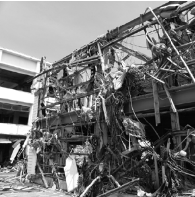
Figure 2. The exterior finish of the steel frame building was washed away, and wreckage was trapped by the structure.
