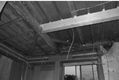
Figure 3. Lack of a beam on the second floor was found after the work started, and a beam was added.
