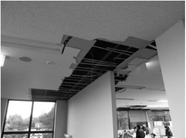
Figure 1. Damage to the ceiling at the top of a partition wall (the Great East Japan Earthquake, 2011) 1)
