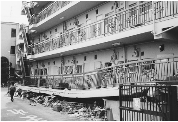
Figure 1. An example of the story collapse of the pilotis part of the ground story
