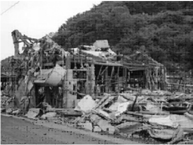
Figure 7. This steel-frame tough building is still standing, but the second floor has been destroyed.
