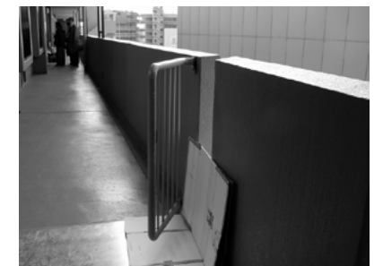
Figure 3. The expansion joint was damaged. The deformation of the balustrade shows signs of very severe shaking.
